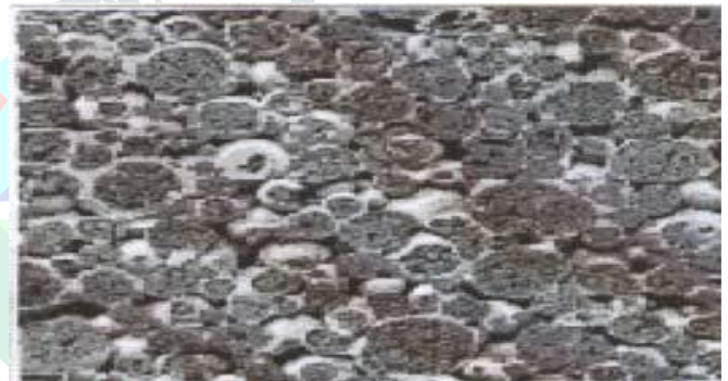
Figure 2: Lightweight aggregate concrete
