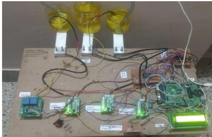
Fig 3: Fuel Display Unit module
