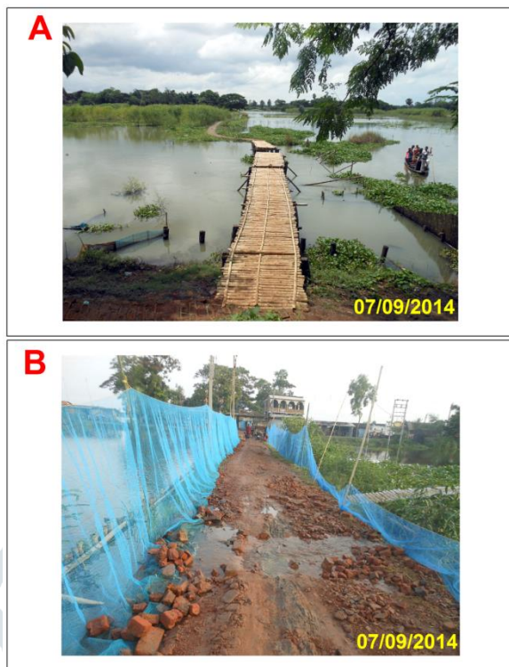
Fig 14 (A) River flow interrupted by local road (B) Surface flow restricted by mud embankment or road
