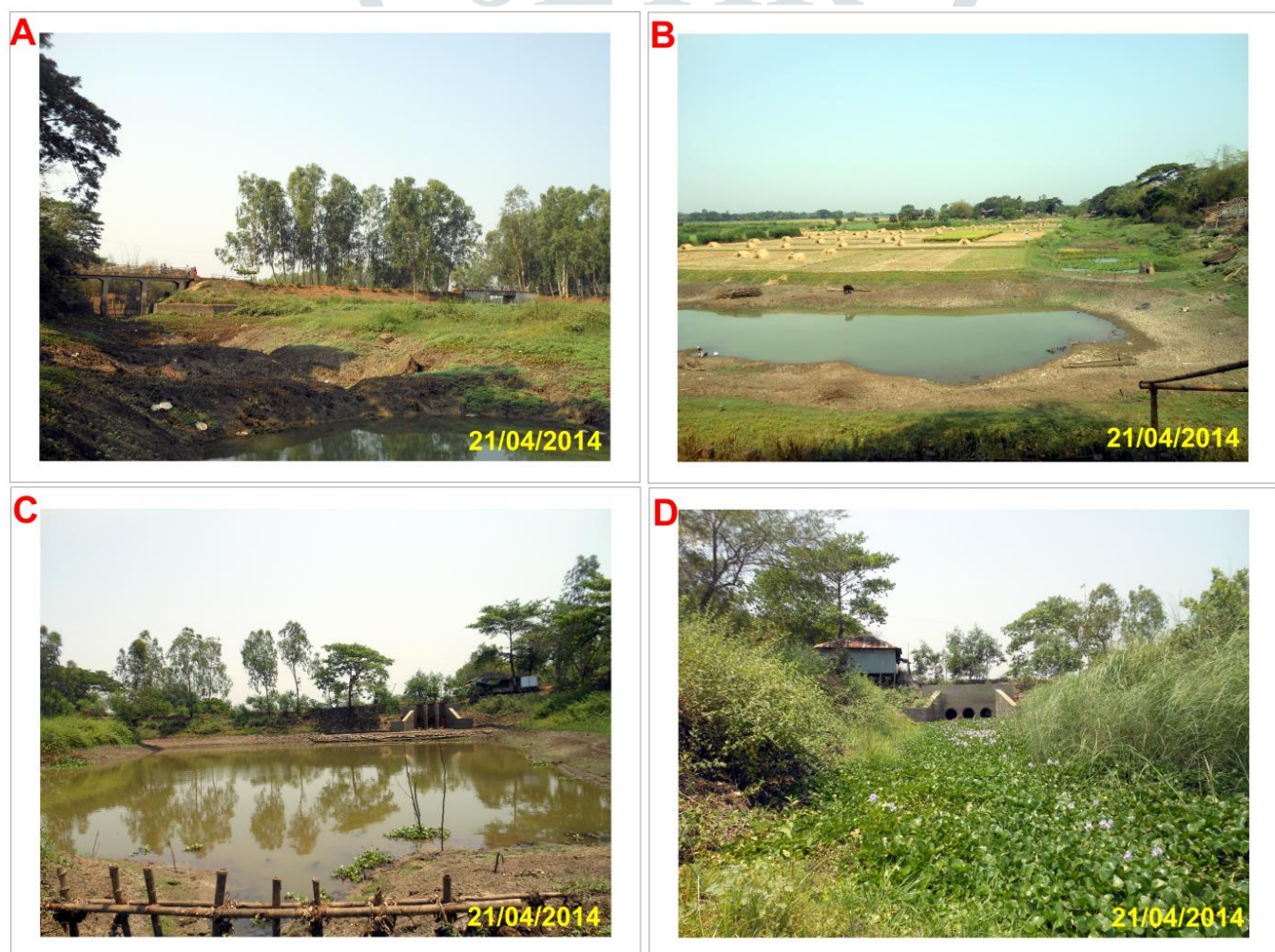
Fig. 16 Flow interrupted by different human activities (A) Small concrete bridge respect to valley (B) Agricultural activity on river bed (C) Small sluice on river valley (D) Small culvert on river valley
