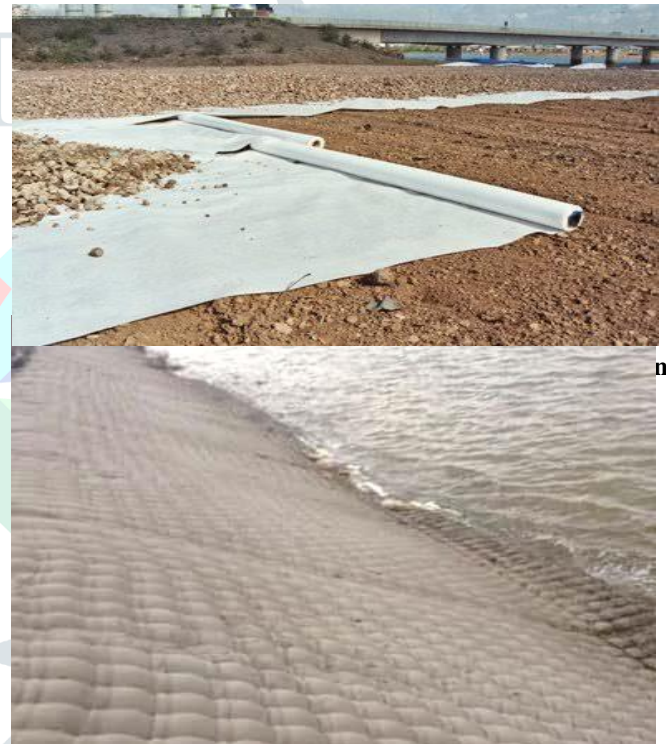
Figure 2: Woven Filament Geotextile used for control erosion at Embankments
