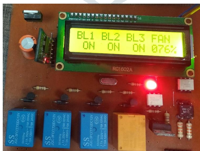
Figure.11 Home automation with display showing the results
