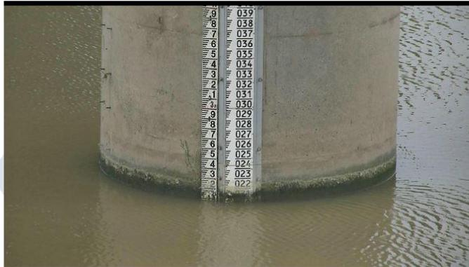
Figure-8. : Level measurement using scale
