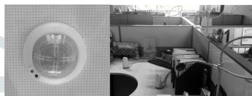
Figure 17 Daylight Sensors in BCA (S. Wittkopf, 2015)
