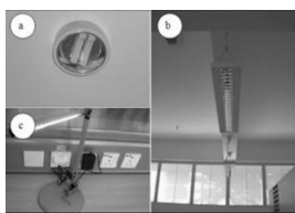
Figure 18 Daylight Sensors in PTM ZEO ( (Poul E. Kristensen, 2007)
