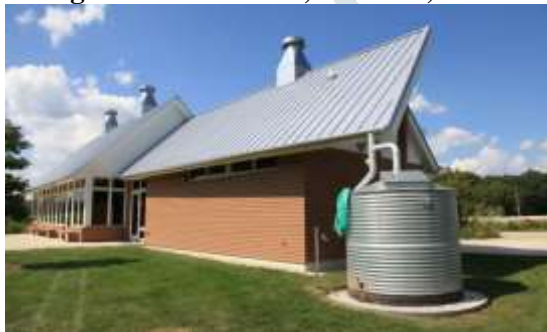
Figure 12: Water harvesting system of a house with green field
