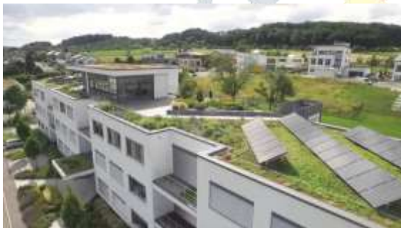
Figure 3: A building with roof gardening and solar panels
