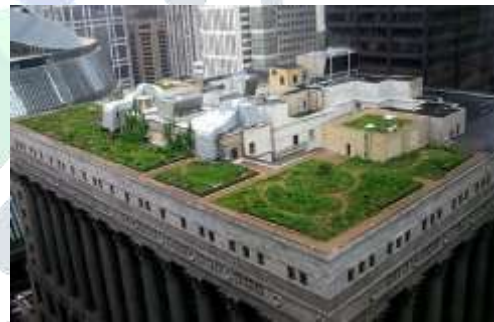
Figure 4: The Chicago City Hall green roof helps cool the building and minimize water run-off
