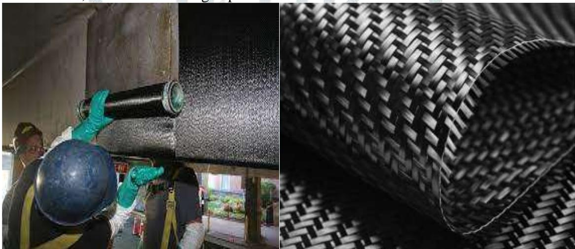
Figure 5: GFRP Sheet Wrapping Technique
