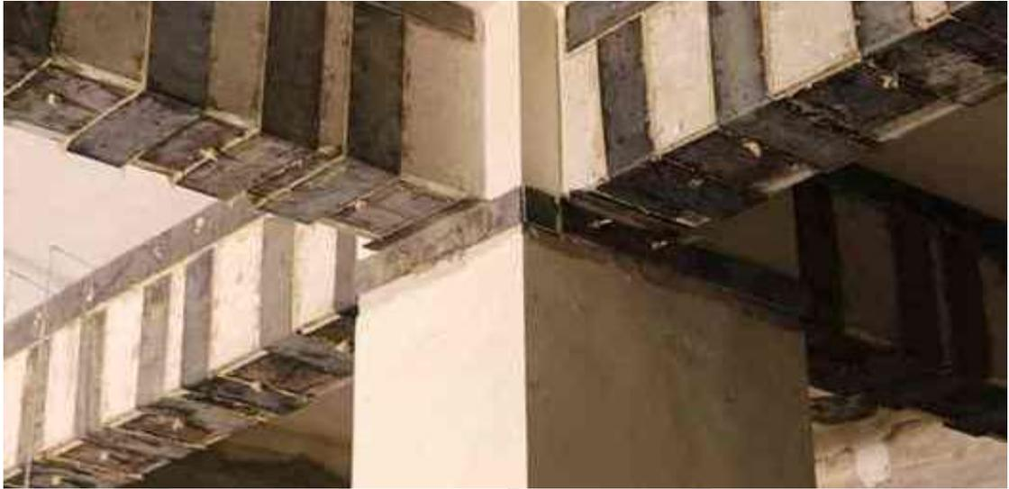
**Figure 6: External Plate Bonding Method**
