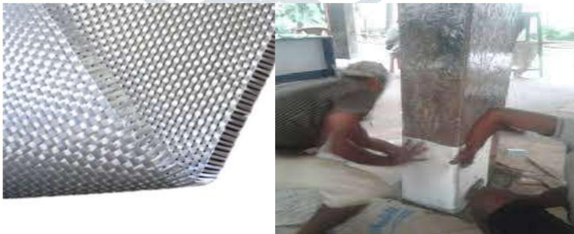
Figure 4: GFRP Sheet Wrapping Technique
