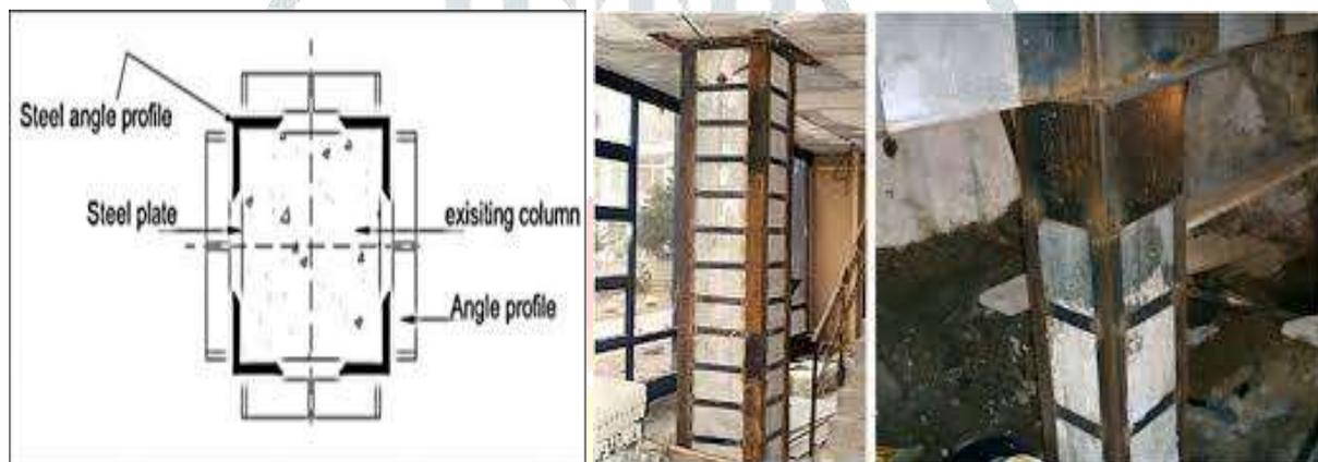
Figure 2: Construction Technique for Steel Jacketing
