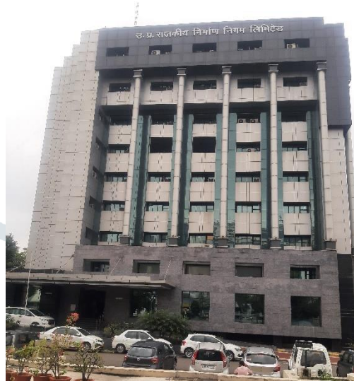
Figure-2 View of building from Mandi parishad road
