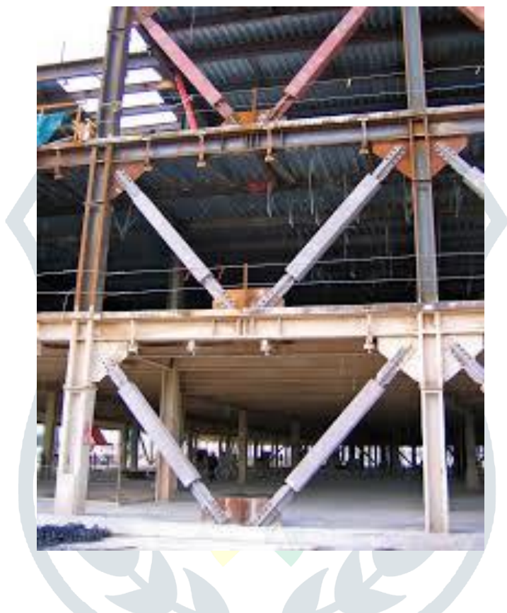
(a) Buckling-restrained brace
