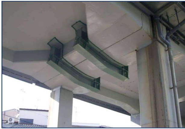
Figure 1.2: Retrofitting of Building
