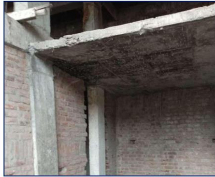
Figure 4.3: Visual Observation of Slab
