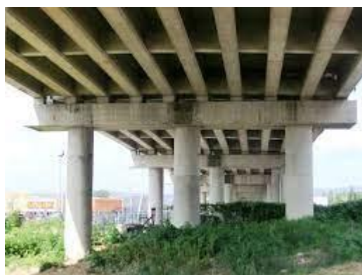
Fig 2:- T Beam Bridge in existence
