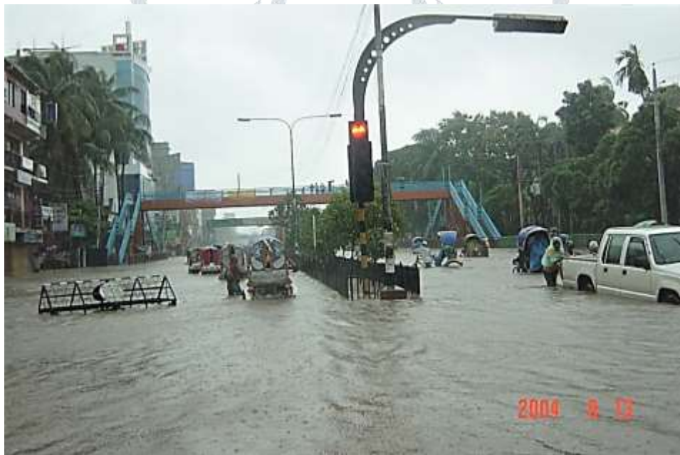
Figure-2: Water-logging at Dhanmondi-27 Crossing on 13 Sept. 2004 (Photo: Author)
