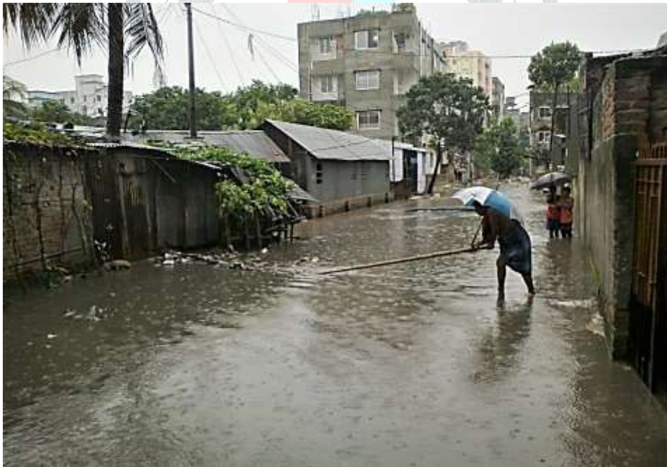
Figure-4: Water-logging for Overflowing an upstream of Kollyanpur Canal between West Shewrapara and South Pirebagh on 11 Sept. 2017 (Photo: Author)
