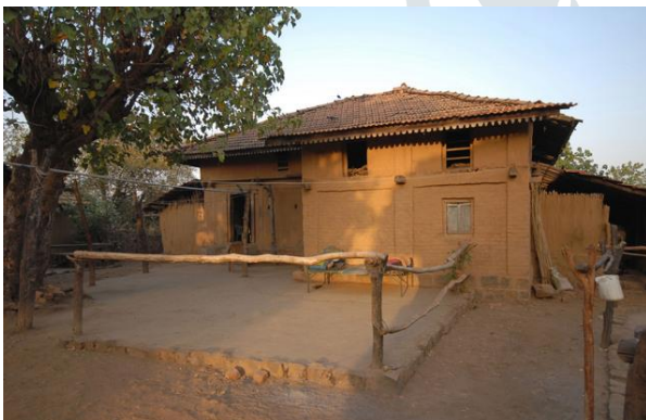
Figure 4 A Bhil Residence Source- Tribes of India
