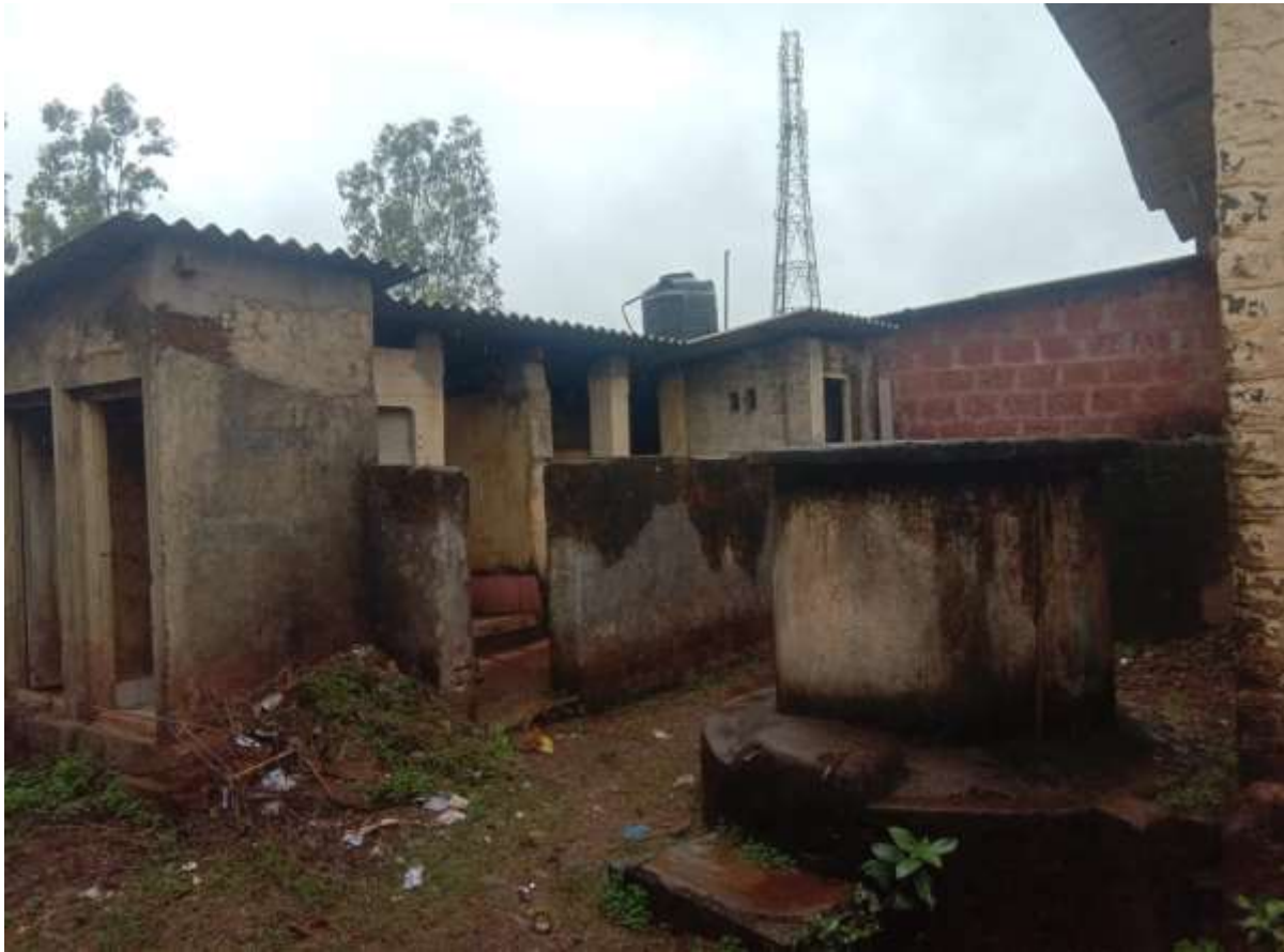
School Toilet Condition
