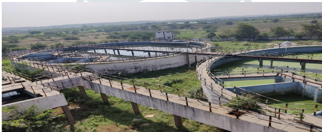
Figure 1 Sewage Treatment plant of capacity 17.5 MLD of Nandurbar City (SBR)
