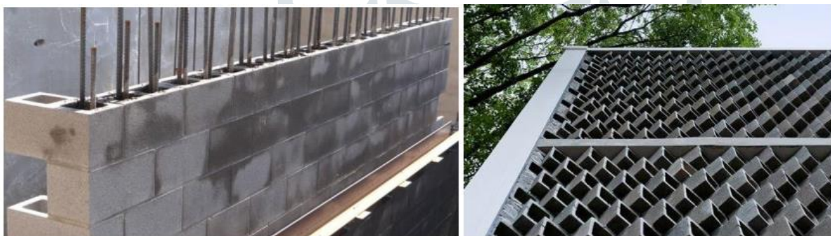
Figure 14 Wall construction made of hollow concrete blocks Source: dezeen,2014
