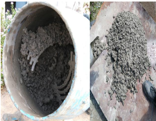
Fig. 3 mixing of concrete
