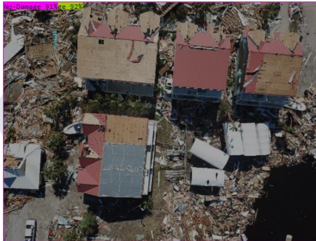
Fig.6.No damage (91%) and Moderate damage (92%) detection
