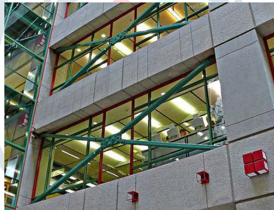
Fig.4 Friction Damper structure
