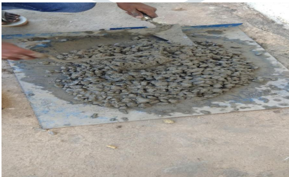
Fig 3.2.2 Mixing of concrete
