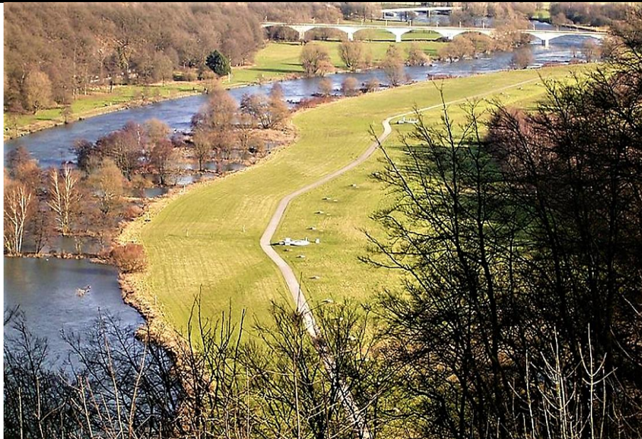
Fig. 6.1 A series of bank filtrate recovery wells along the Ruhr river in Hattingen (Germany). Source: VINCENTZ (2008)
