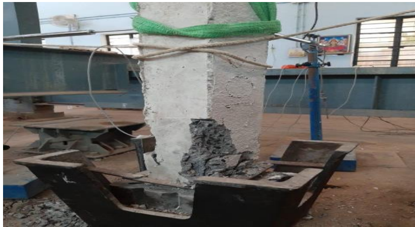
Fig 6.0: Column with 10mm steel as longitudinal rebar's. SPECIMEN 2
