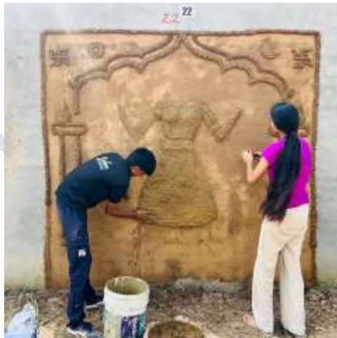
Fig. 8: Plastering of the wall with cow dung.
