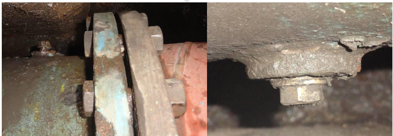
Figure 6 replacement of old dummy by SS material
