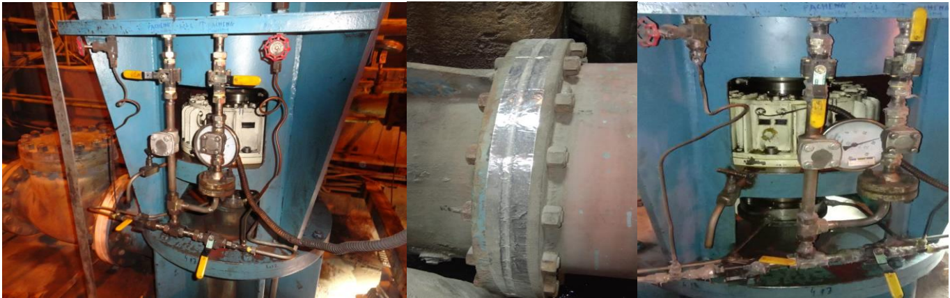
Figure 7 replaced with all new o rings, gasket in sealing system
