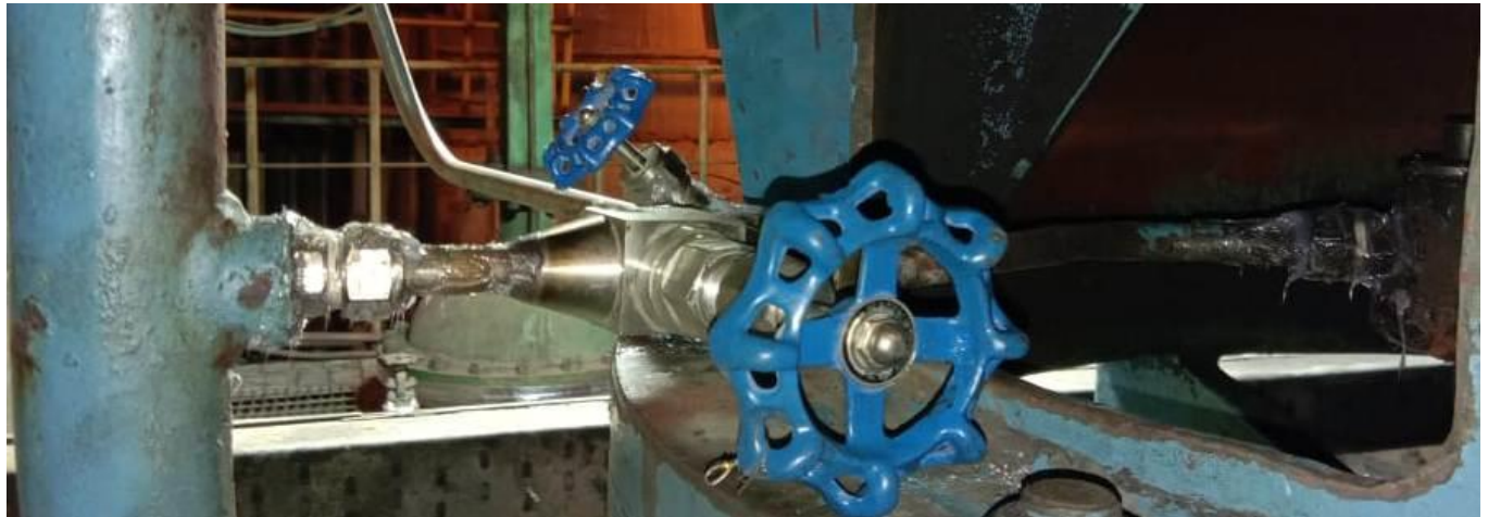
Figure 4 replacing connector joint to welded valve and fitting.
