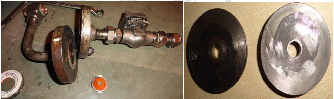
Figure 5 modification of CEP discharge make up line orifice.
