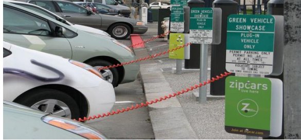
Fig.1 EV charging station
