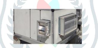
In order to maintain indoor air quality, air handlers commonly have provisions to allow the introduction of outside air into, and the exhausting of air from the building. In temperate climates, mixing the right amount of cooler outside air with warmer return air can be used to approach the desired supply air temperature. A mixing chamber is therefore used which has dampers controlling the ratio between the return, outside, and exhaust air.
