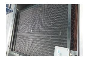
AHU Cooling coil used Refrigerant as direct expansion system. Refrigerant temperature at direct expansion system can be low as 2'C.
