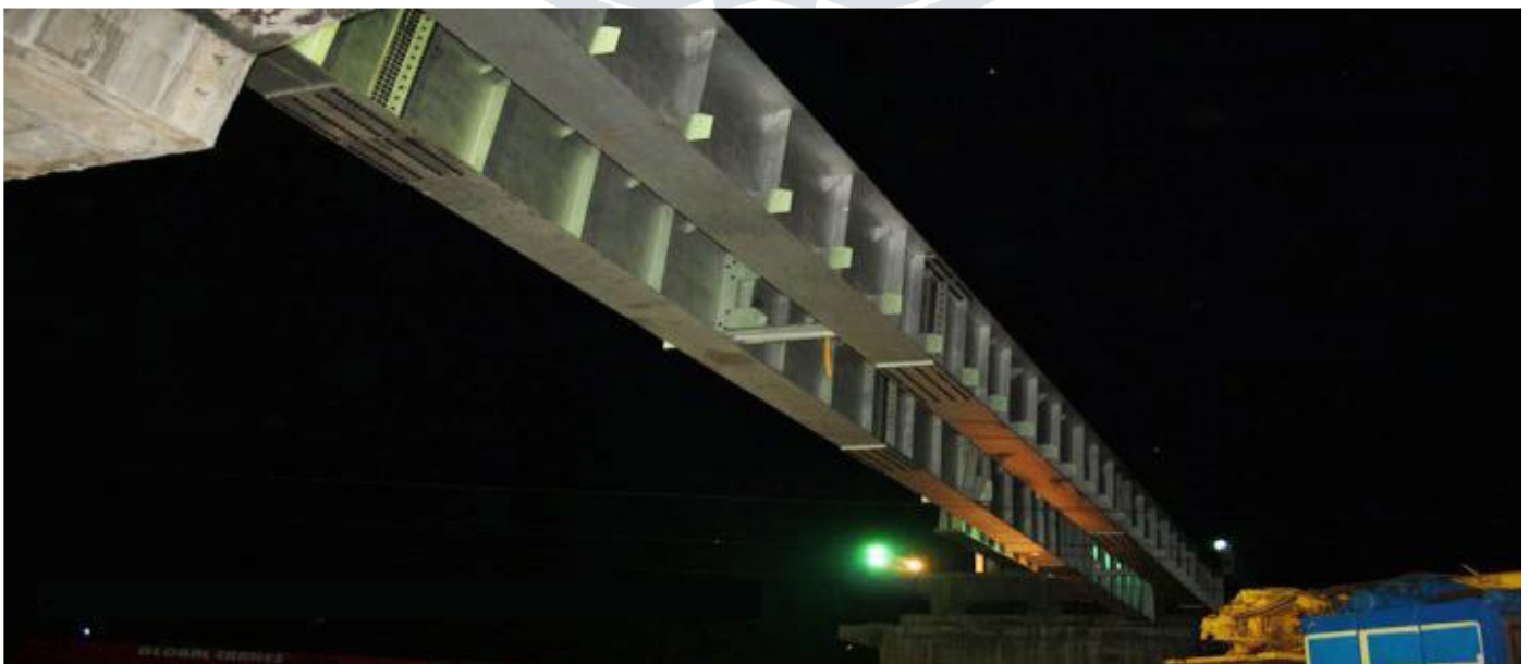
Fig -2: I section girder on ROB.
