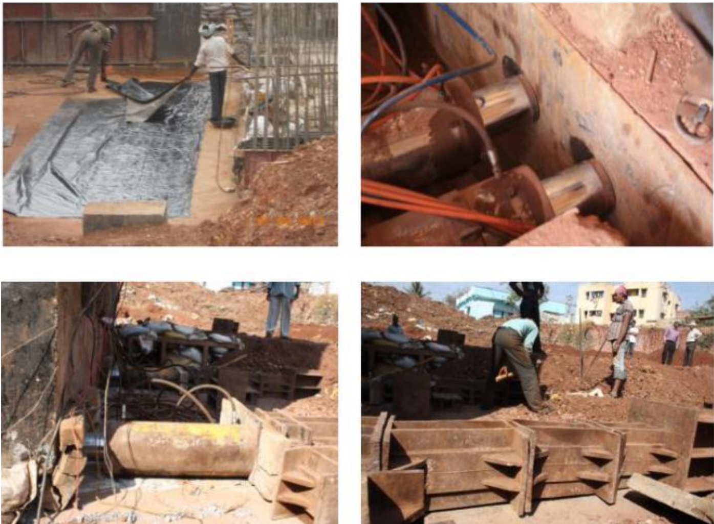
Fig 5: Pushing of Box Segment with help of Piston.
