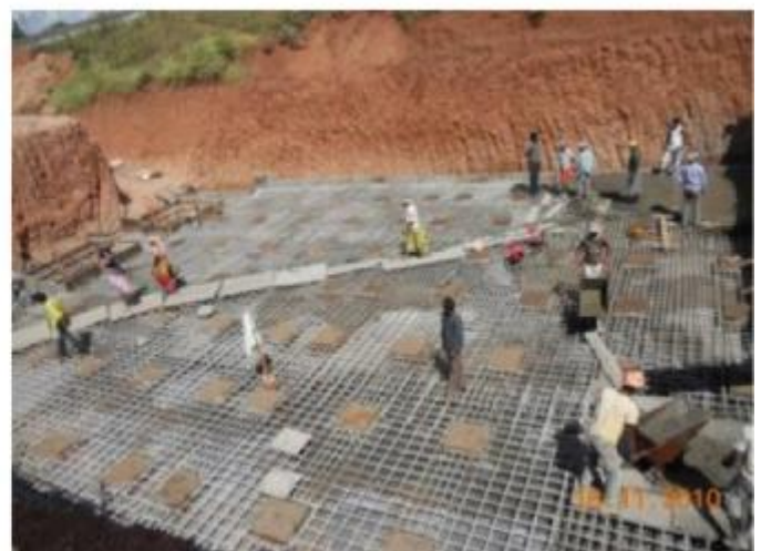
Fig -4: Foundation of road in Box Pushing in RUB.
