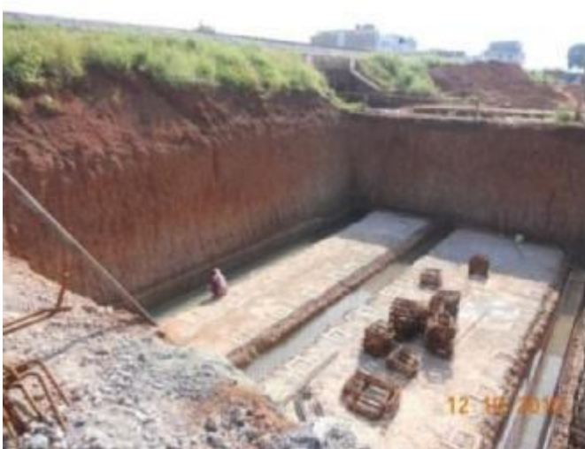
Fig -4: Foundation of road in Box Pushing in RUB.
