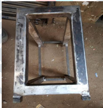
Fig.1 Fabrication of Frame
