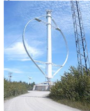
Fig.1: Vertical Axis Wind Turbine
