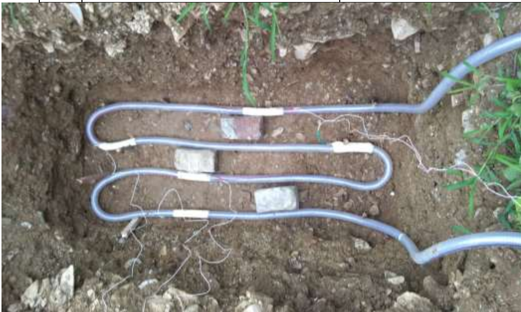
Figure 3.2: Corrugated profile pipe setup in ground
