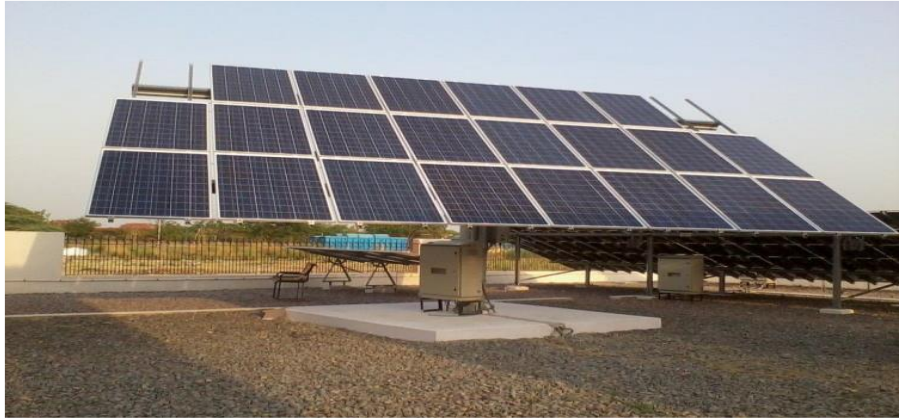
Fig. 6: Multi-Crystalline PV system (tracker)
