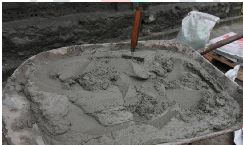
Fig 2: Cement Mortar [F4]
