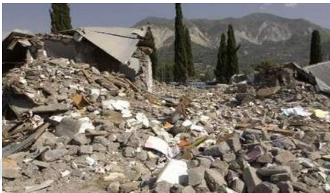
Figure 3 Damage to Stone Masonry Building in Kashmir Earthquake 2005
