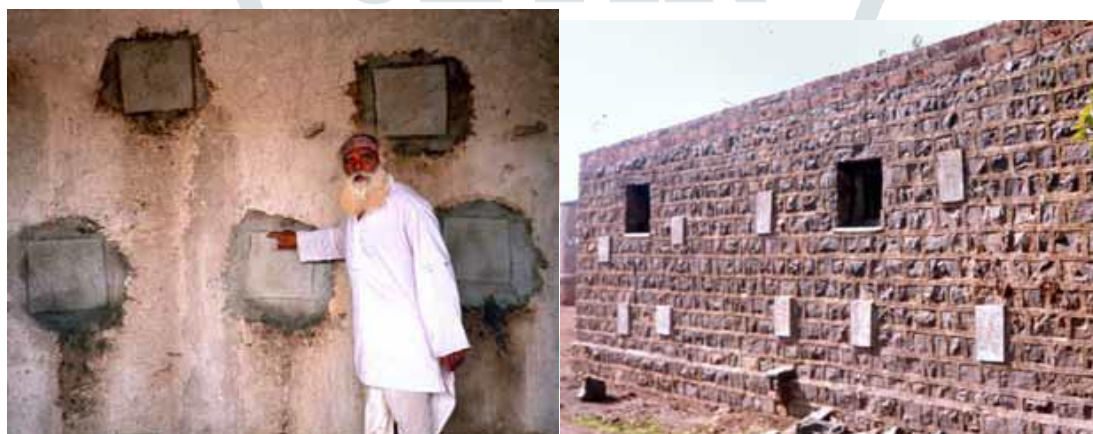
Figure 10 Examples of completed through-stone retrofit projects in Maharashtra, India
