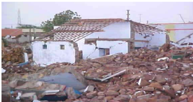
Figure 2 Damage to Stone Masonry Building in Bhuj, Gujrat Earthquake 2001
