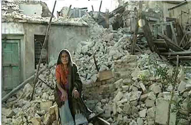
Figure 4 Damage to Stone Masonry Building in Maharastra
