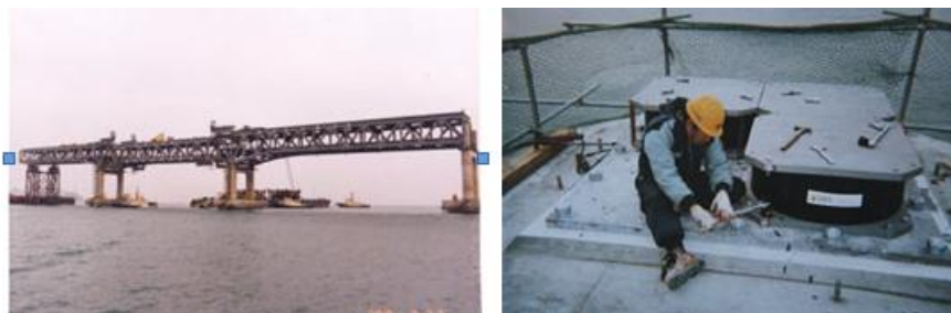
Figure 4 Kwangan Bridge with Lead Rubber Bearing
