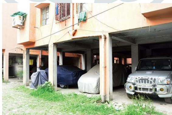
Fig.1.1 Open Ground Storey (Reference: 10)
