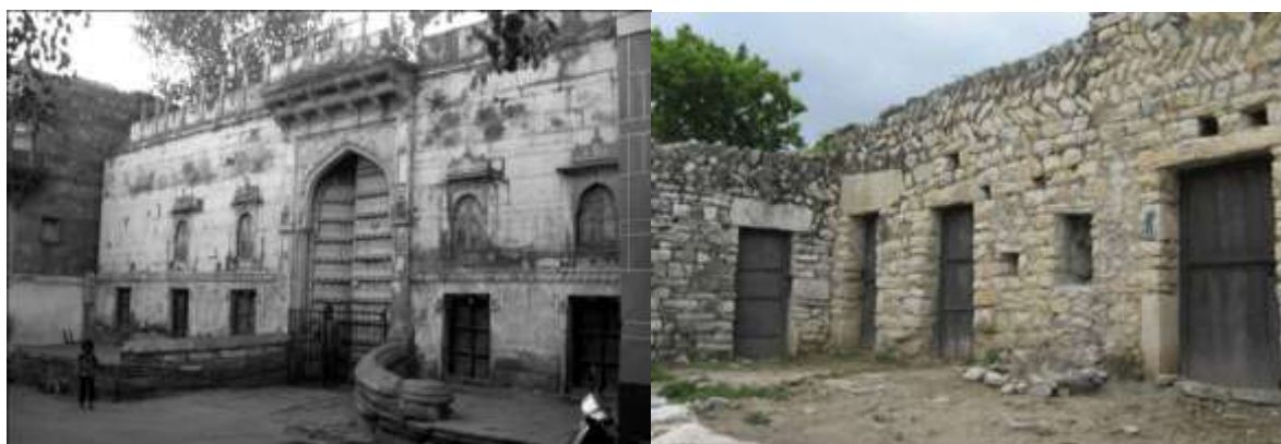
Figure 2: Stone masonry construction in Rajasthan: a) a typical stone masonry house in Jodhpur, and b) a typical rural house in a village of Jodhpur
