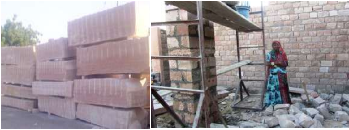
Figure 3: Stone masonry construction: a) Un-dressed stones for construction, and b) Stone masonry construction in Jodhpur, Rajasthan, India
