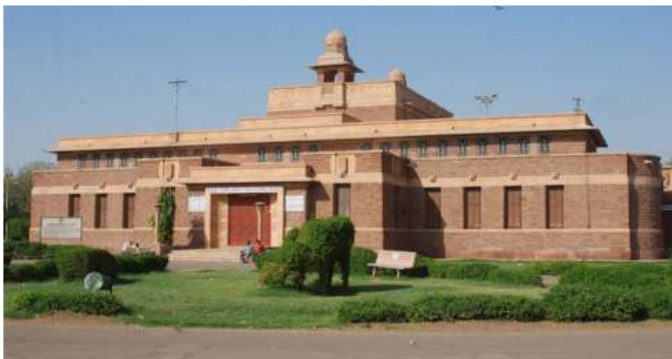
Figure 1: Traditional stone masonry building in Jodhpur, Rajasthan
