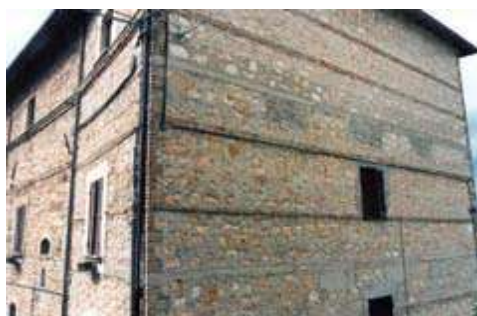
Figure 9: Seismic-strengthening techniques in Italy: installation of new steel wall ties
