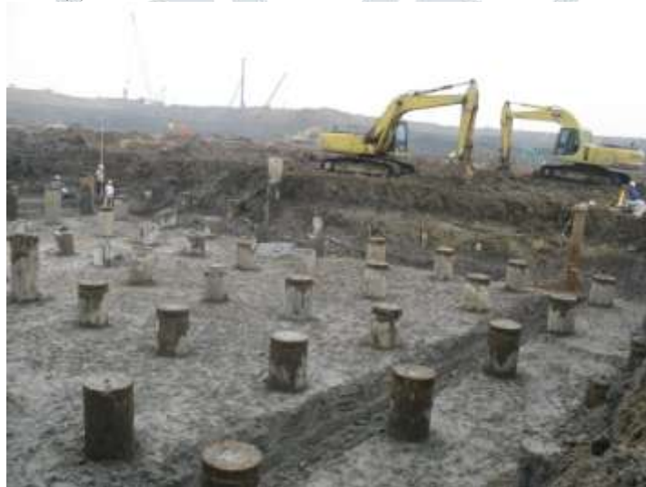
Figure 1 showing pile foundation
