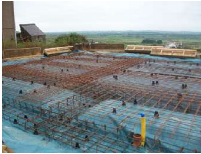
Figure 2 showing raft foundation
