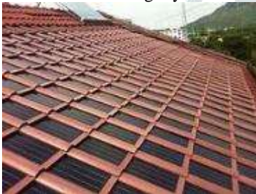
3.1.5) Solar roof PV tiles [2]
