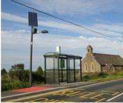
3.2.2) Solar Street light at the bus stop
