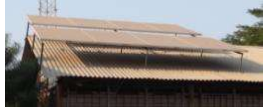
3.1.7) Pitch roof solar panel installation (Belgaondhaga, Nashik)
