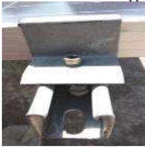
3.1.4) Slide in clamps and locked modules at ends of rails
