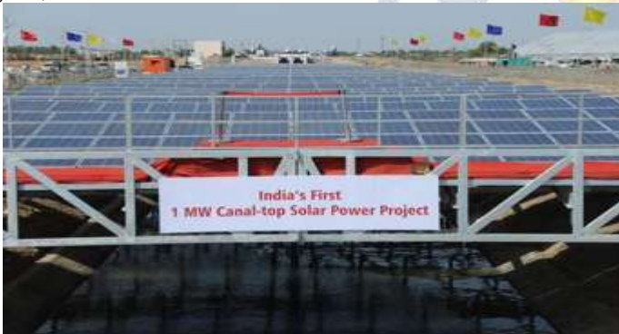
3.15.1) India's first 1MW Canal-top solar power project
