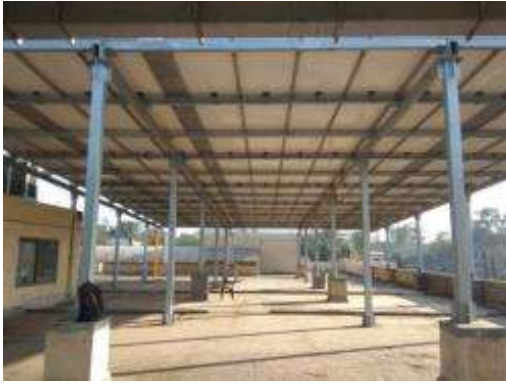
3.1.3) Beam structure- Galvanised hot dipped steel structure
