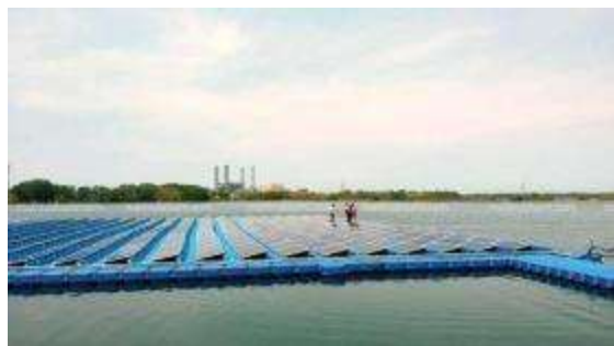
3.16.2) India's Largest 100 KW System, Kerala
