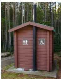
Figure 7 - solar chimney
