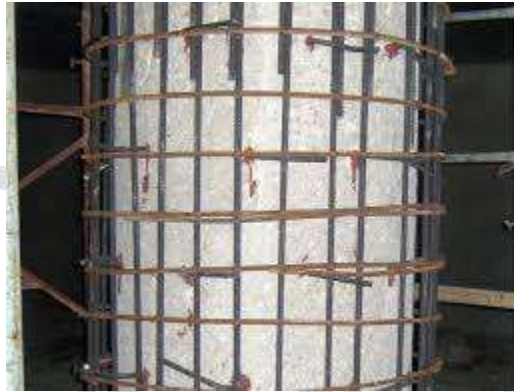
Figure 2. RCC jacketing of piers
