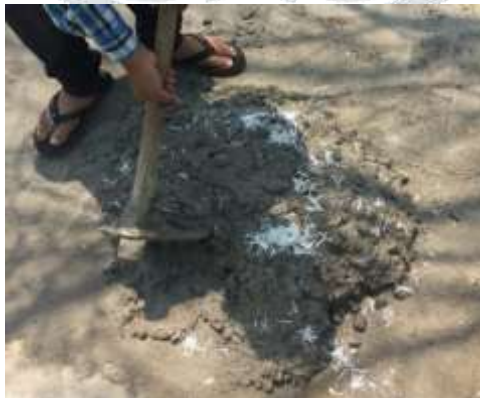
Figure 4: Shows Mixing of Concrete
