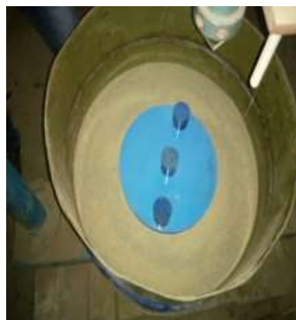
Figure 3 Placing of footing plate on compacted soil
