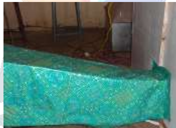
Fig.5 Duct of reducing cross- section
