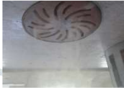
Fig.14 Air distribution pattern through 12 0 ceiling Swirl Diffuser
