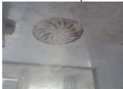
Fig.12 Air distribution pattern through 10° ceiling Swirl Diffuser
