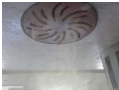
Fig.13 Air distribution pattern through 11 0 ceiling Swirl Diffuser
