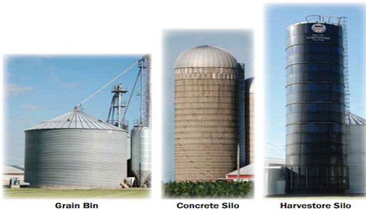
Fig. 1 grain bin, concrete silo, harvestore silo
