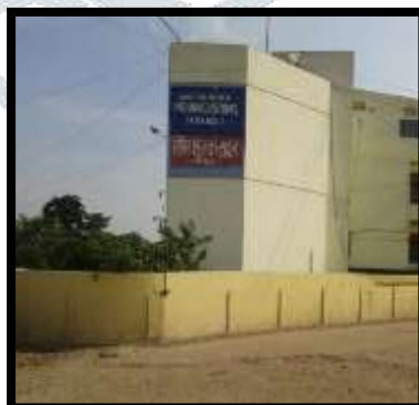
Figure-2 : Custom Office Bridge
