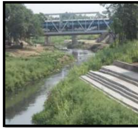
Figure-4 : Railway Bridge at Islampur, Raxaul
