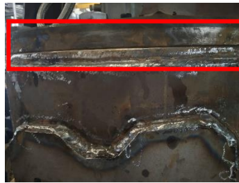
Fig 2.2: Welding of base plate with supports
