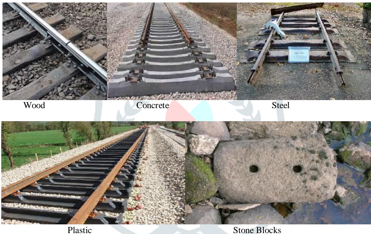
Figure 4: Different types of sleepers [1]
