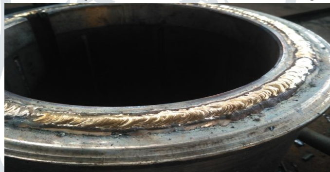
Fig.9: Completion of welding on sleeve neck
