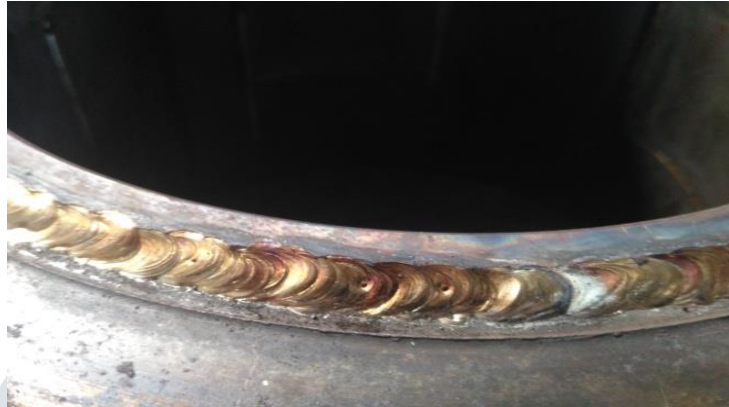
Fig.8: Partial welding on sleeve neck
